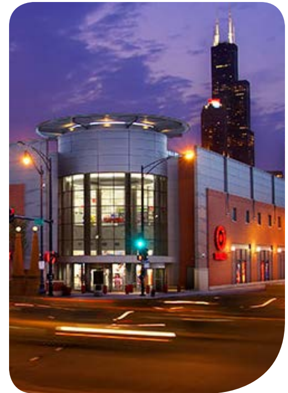
At our West Loop store in downtown Chicago, we've installed white roof membranes that reflect sunlight to lower our cooling needs, plus LED lights in exterior signs.
