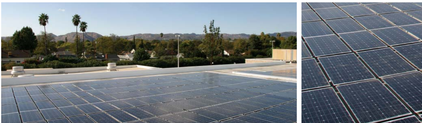
Solar roof panels harness the sun's energy at a Los Angeles Target store.
